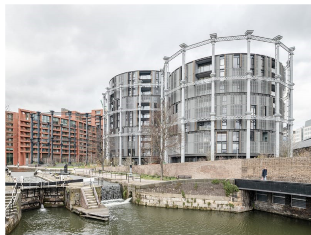
Figura 12. Ruin or Rust: King's Cross Gas Holders, 2020.
