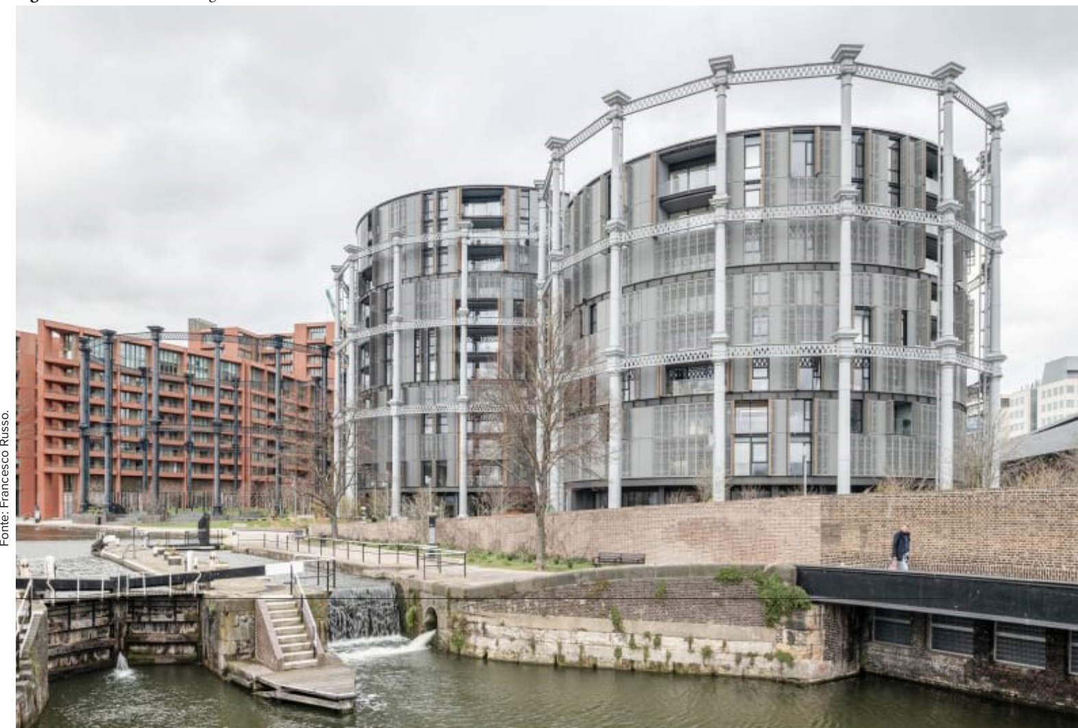
Figura 12. Ruin or Rust: King's Cross Gas Holders, 2020.
